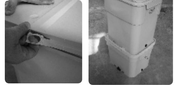
Insert a 1/2" **barbed, straight fitting** and connect the Controller to the Reservoir with the 1/2" **Blue Tubing**. Measure before cutting the tubing to avoid cutting it too short and the tube kinking.
