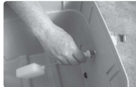
Secure the Float Valve from the outside of the Controller with the brass nut. Coat the remaining threads with the Pipe Thread Compound and screw on the brass 1/2" barbed hose fitting.
